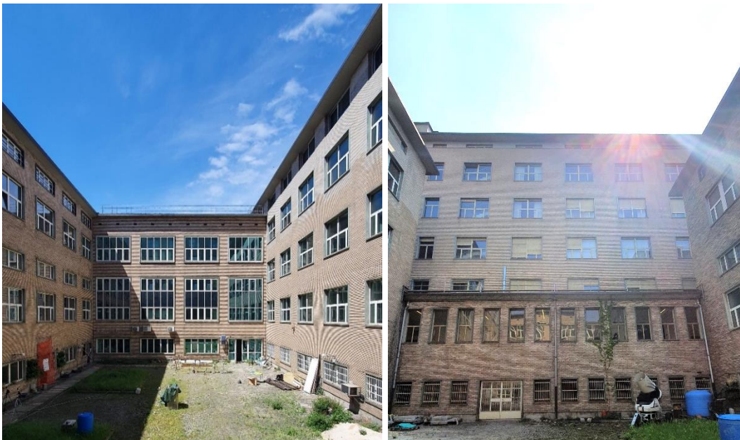
Figure 52. Photograph of the courtyard used as case-study
