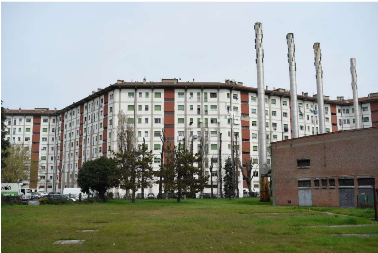
Figure 2 - View from the district heating plant in Pilastro and a part of the social housing dwelling
