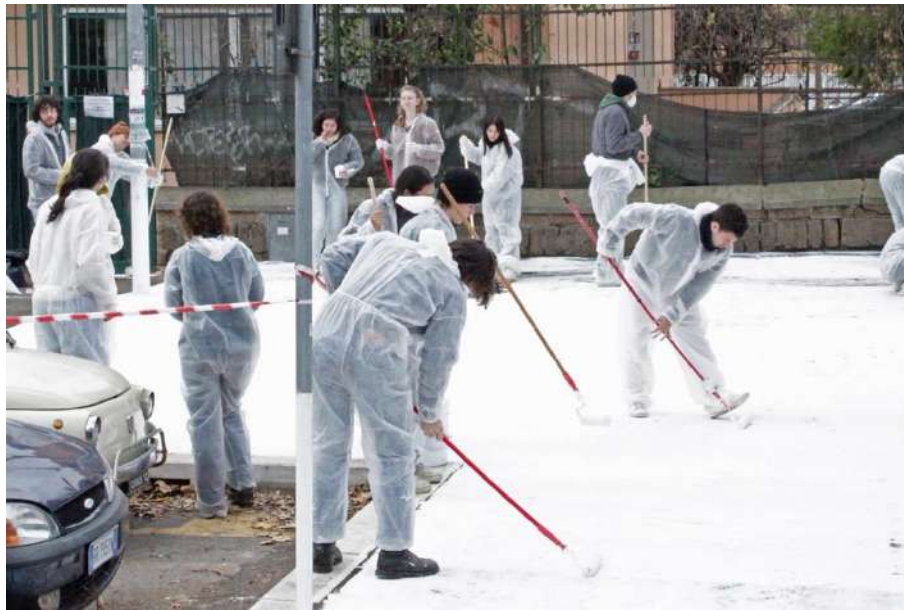
Figure 6: “Marciapiede Fresco”, the open construction site to test the Cool Materials technique. (Largo da Vinci-Rome, credits: Fabrizio D’Angelo, 2023).
