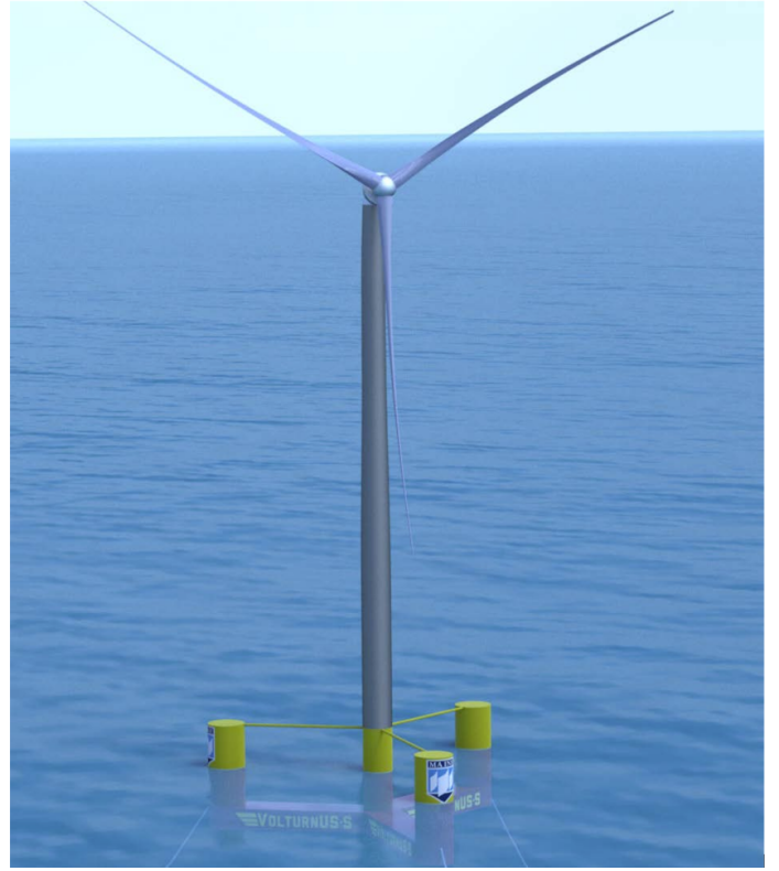
FIGURE 1: UMaine VoltturnUS-S platform designed for the IEA-15-240 RWT system [7].
