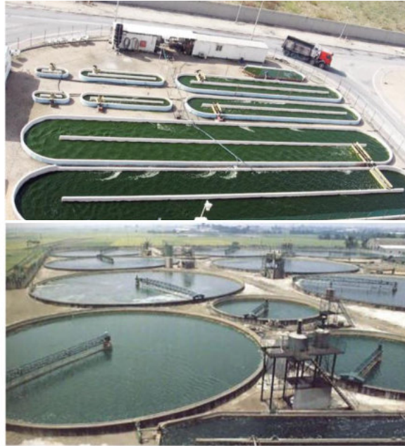
Figure 5: Examples of open ponds systems. Raceway on the upper image from U.S. Department of Energy National Renewable Energy Laboratory. In the lower photo a circular open pond system.
