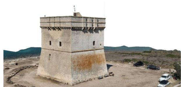
Figure 14. Photorealistic textured 3D model of Torre Chianca in Porto Cesareo (LE). Mesh composed of 902’132 faces and 451’079 vertices.
