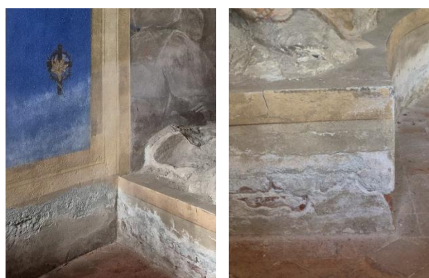
Figure 5. Detail on Chapel XVI's degradation processes
