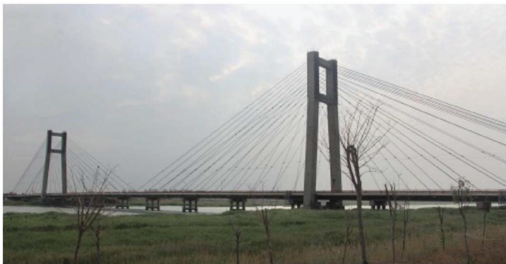
Figure 3. View of the Yonghe Bridge, Tientsin, China.
