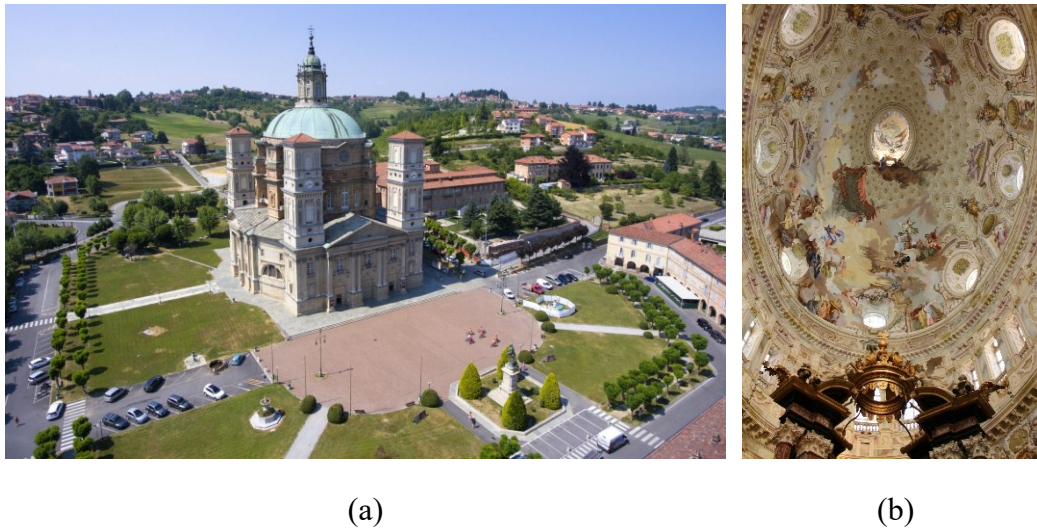
Figure 5. 19. Geometric and structural overview of the Sanctuary of Vicoforte : (a) aerial view of the Sanctuary and its immediate surroundings; (b) Internal view of the oval masonry dome.
