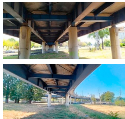
Fig. 2. View of the underside of a generic 4-beams and a 2-beams viaduct.
