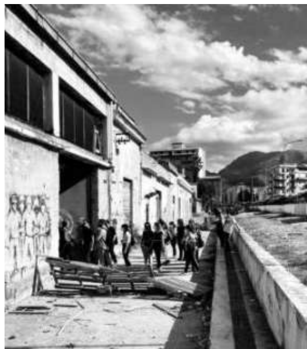
Fig. 5. Palermo, The former Pensabene factory on via Chiaramonte , inspection with students (photo S. Oddo).
