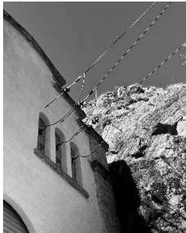
Fig. 3. Campliccioli power house, 1924-1930, transmission lines (photo by the author).
