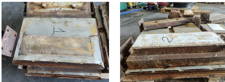
Figure 5 Multi-directional Teflon bearing - lower plate (left) and upper plate with Teflon sheet (right)
