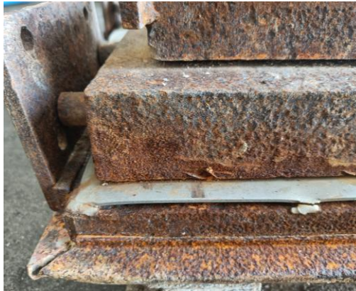
Figure 9 Incomplete welding of the steel plates
