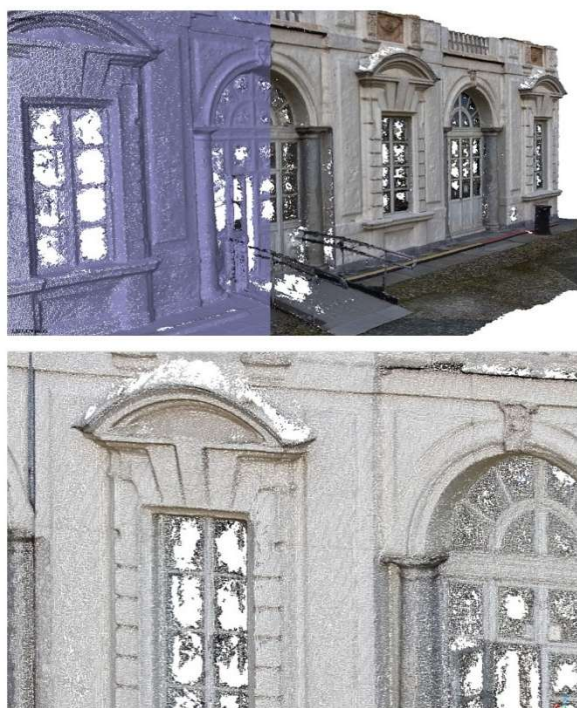
Figure 11. Example of the level of detail of the 3D point cloud based on the GNSS-Ph approach
