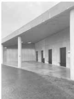
From exterior to interior
