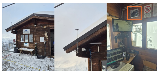
Figure 1. The Prali LC GNSS station at approximately 2200 m elevation: (left) building with antenna mounted on a pole, (centre) detail of the LC antenna installation, (right) indoor hardware including the u-blox ZED-F9P receiver and Raspberry Pi in a weather-resistant enclosure (highlighted).
