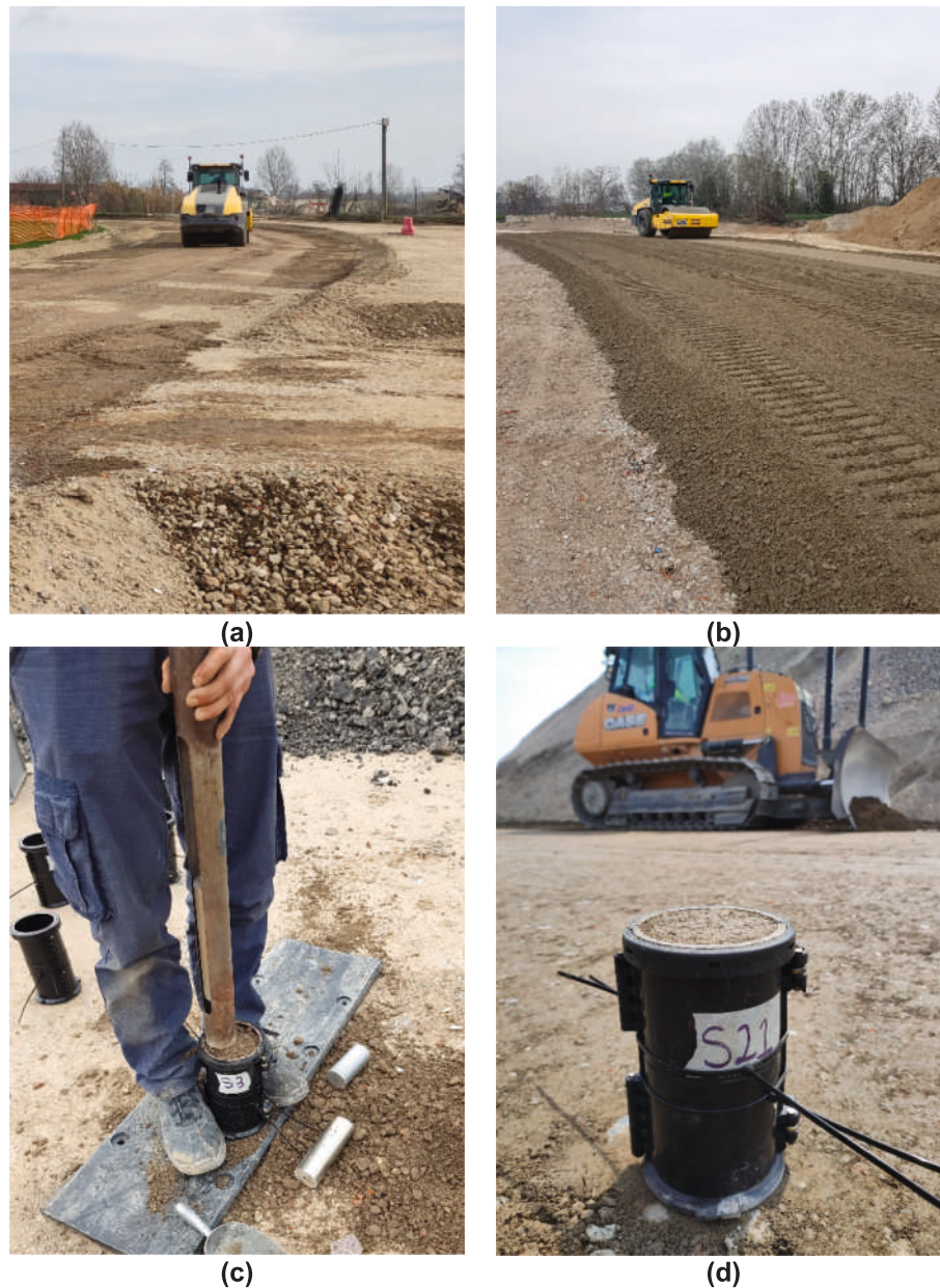
Fig. 8. Construction phase: (a) compaction of subgrade, (b) formation of the CS-NAT subbase, (c) preparation of cylindrical samples for laboratory characterisation, and (d) compacted specimen in the plastic split mould.
