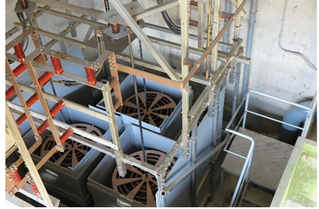
FIGURE 3 | Refurbished power dissipation system.
