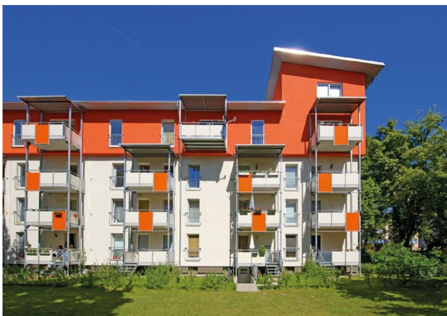
Fig. 5 – 192 Shoreham Street, Sheffield, 2012, progettisti Project Orange (ph. J. Hobhouse, tratta da Roofscape Design cit.).
