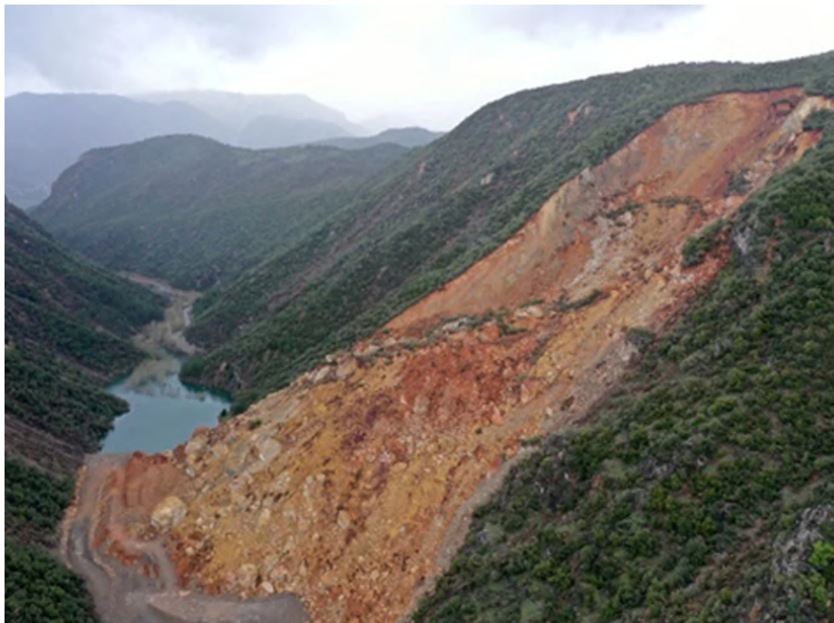
Figure 2-17 Landslide caused by earthquakes in İdilli, Turkey (Kocaman et al., 2025).
