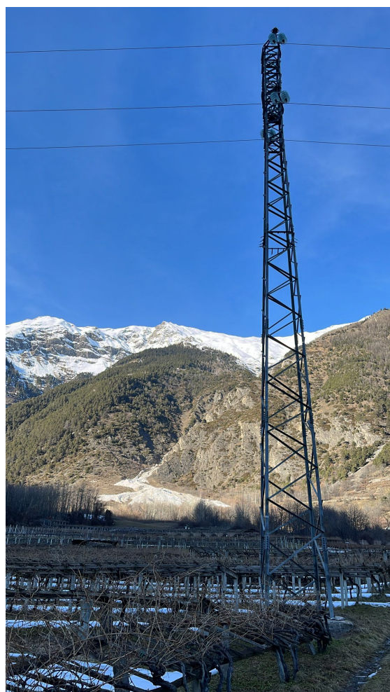
Figure 10. Transmission tower under investigation.
