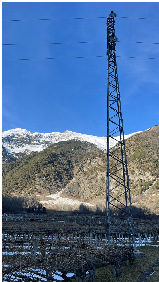
Figure 10. Transmission tower under investigation.
