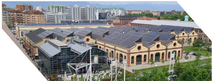
Fig. 1. View of the photovoltaic system installed on the rooftop of the Politecnico di Torino canteen.
