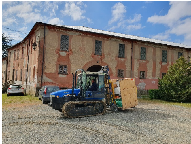
Figure 74: Moving the main body using the forklift mounted on the back of a tracked vehicle.
