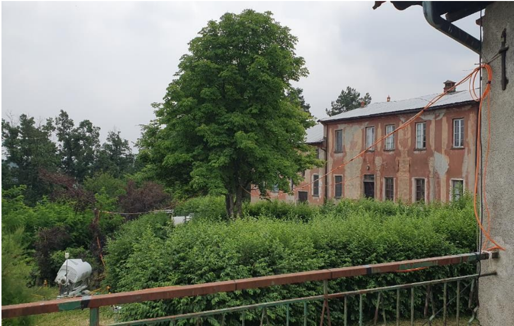
Figure 88: Positioning of the overhead cables between the balcony and the building where the PC is located.
