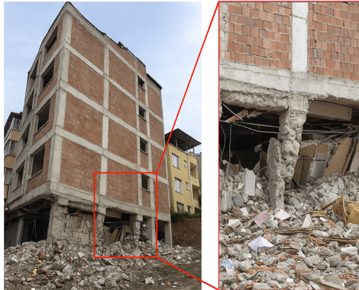
Figure 1.4: Example of soft-storey mechanisms.
