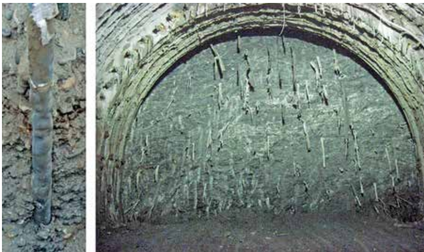
Fig. 10 – PERGround® bar removed after injection (left). Tunnel face improved by means of PERGround® (right).
