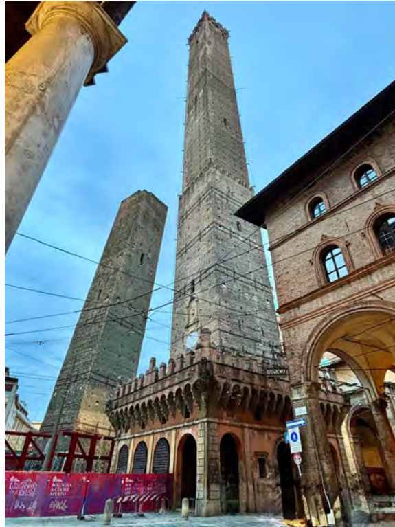
Figure 1. The Garisenda (left) and Asinelli (right) Towers in Bologna.
