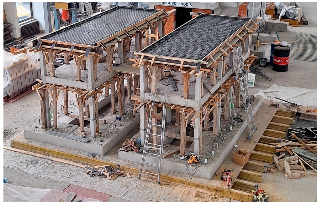
Figure 3. Building of the RC structure.
