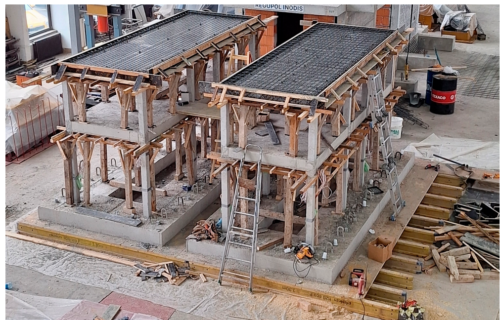
Figure 3. Building of the RC structure.
