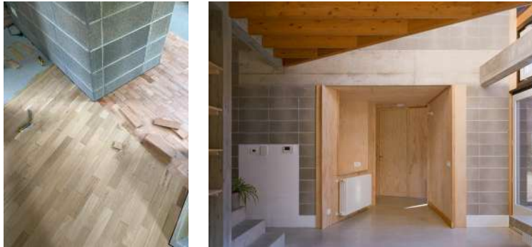
Casa BM, the investigation of semi-finished product stocks and economical building materials oriented the project. Wood panelling, shelving and fixed furnishings were all produced on site with limited tools and visible fixings. Photo: ErranteArchitettura / Luca Bosco
