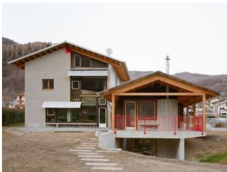
Casa BM, the new composite façade on the south front of the existing building, realised in collaboration with a local joinery company. Photo: Luca Bosco
