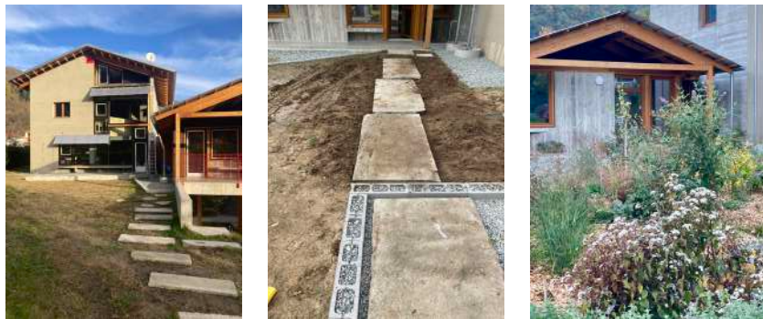
Casa BM, the cataloguing and reuse of materials from the site and its immediate surroundings. Steps from the demolished staircase of the original building define the paths around the house, while stone slabs from a nearby ruin mark the entrance area. The garden forms a patchwork of 'domestic' and 'wild' plants—some purchased, some preserved, others arrived by chance or found along the roadside. Photo: ErranteArchitettura
