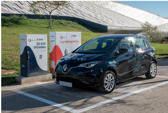
FIGURE 7. UC7 at zaragoza demonstration site: electronic and cooling system cabinets and charging area.
