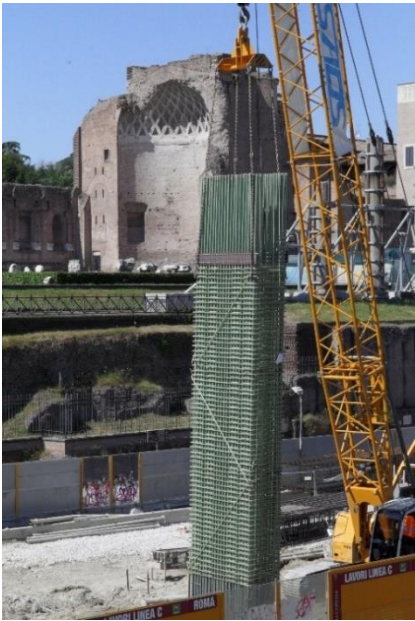
Figure 19. Installation of a GFRP cage
