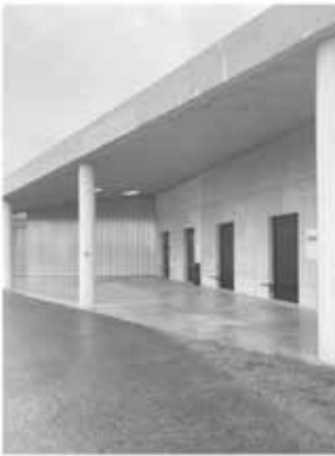
From exterior to interior
