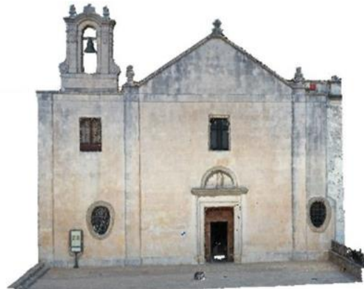
Fig. 3. Point cloud of the external structure generated by photogrammetric survey from UAV.
