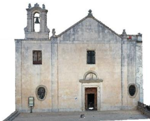
Fig. 3. Point cloud of the external structure generated by photogrammetric survey from UAV.
