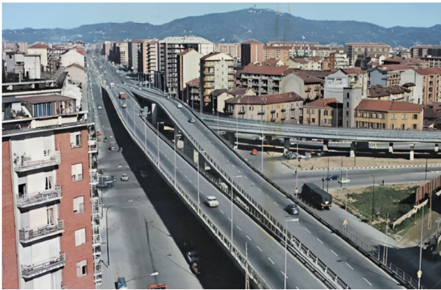
FIGURE 1 A view of the multilevel Corso Grosseto viaduct.
