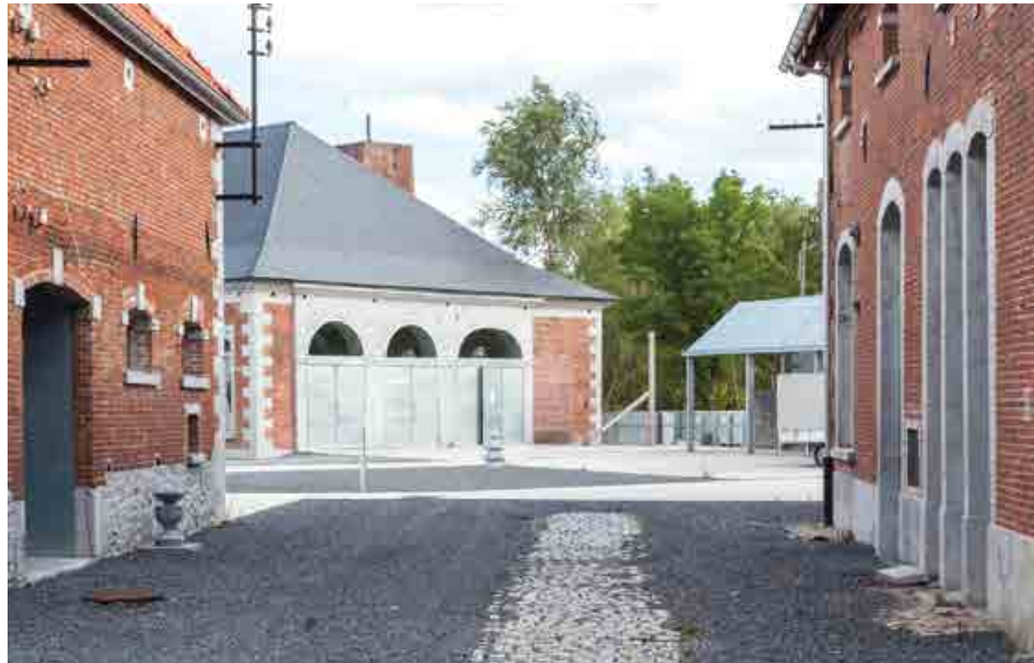
↓ The Grande Scierie seen from the pavilions reused as a cafeteria (left) and museum (right) / © Tra Architetti
