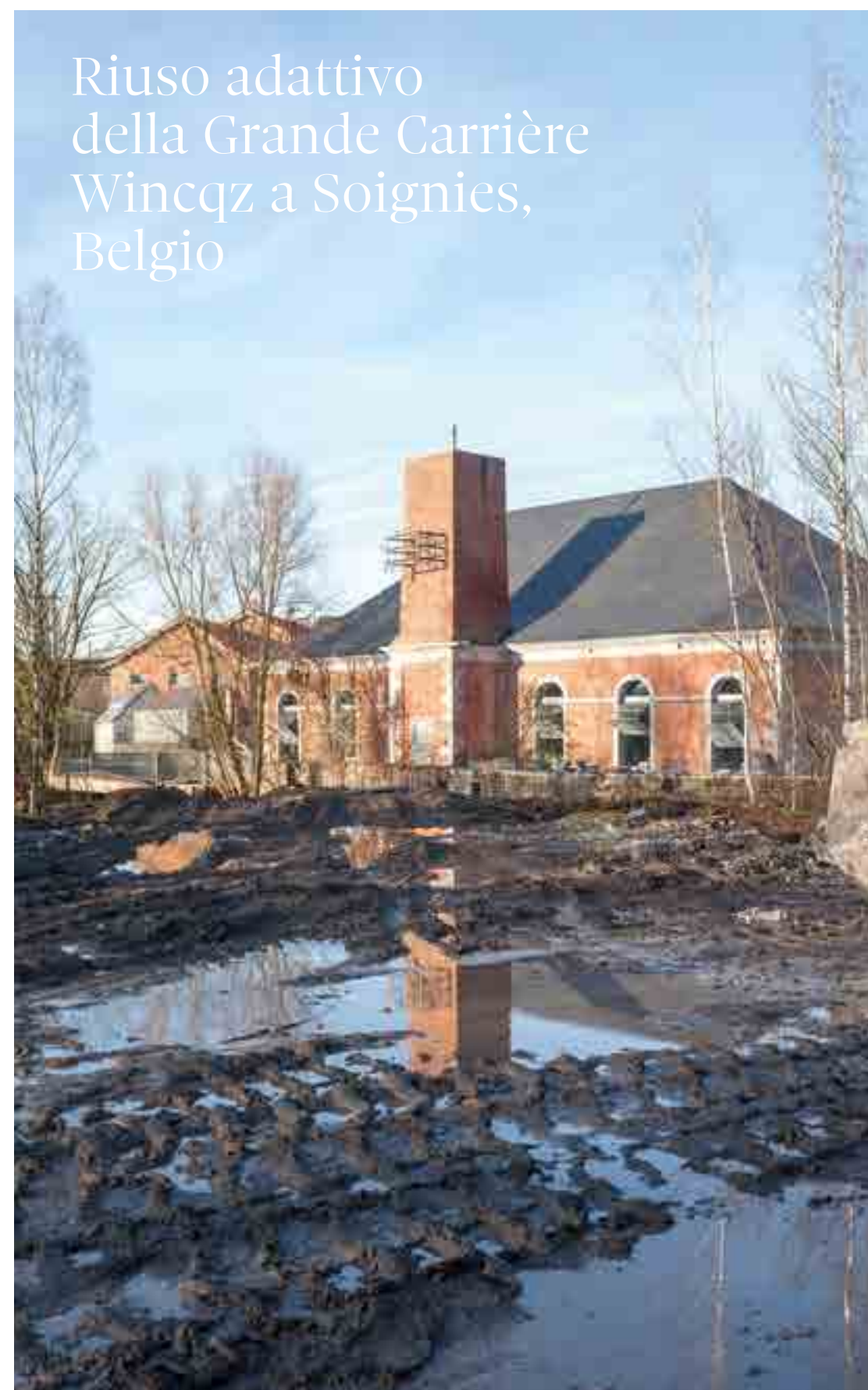
↑ The Grande Scierie as seen from the active mining site / © Tra Architetti
