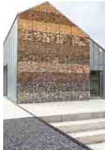
↑ Façade of the new workshop pavilion: rock library of different Wallonian stones worked in pieces / © Tra Architetti
