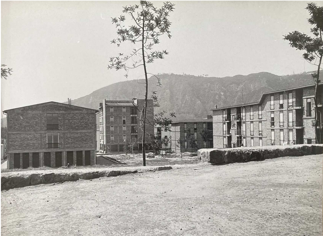
Figure 3. INA-Casa neighbourhood in Soccavo, Naples, Italy. Photograph, 1950s (date unknown). Luisa Anversa Papers.
