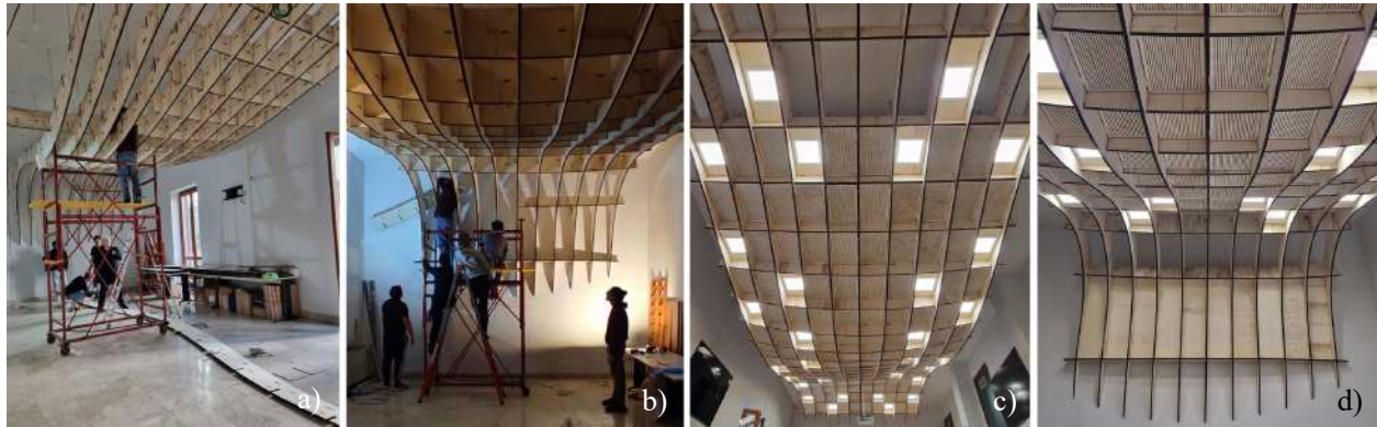
Figure 12. a) Installation of longitudinal beams. b) Fitting of transversal elements within the waffle grid. c) Completed structural framework. d) Realized Schroeder diffuser integrated into the rear section.
