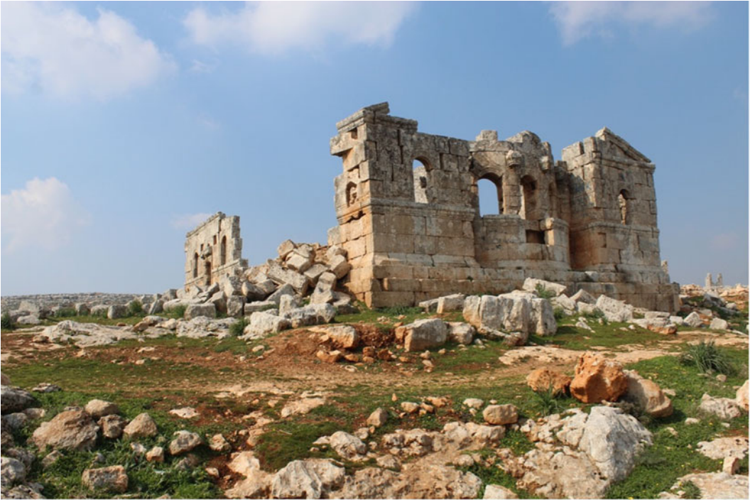
Figure 1. Documentation of damages on Banqusa archaeological site, Idlib, Syria, following the earthquake on February 6, 2023.
