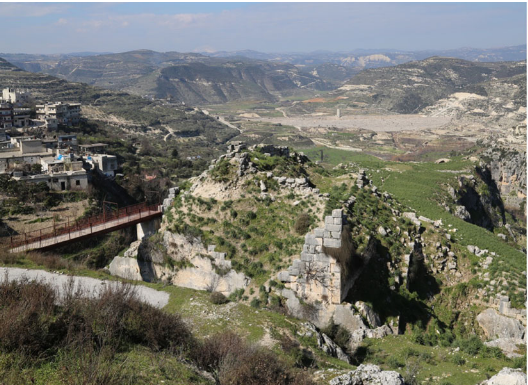
Figure 2. Documentation of damages on Alshoqor Castle, Idlib, Syria, following the earthquake on February 6, 2023.
