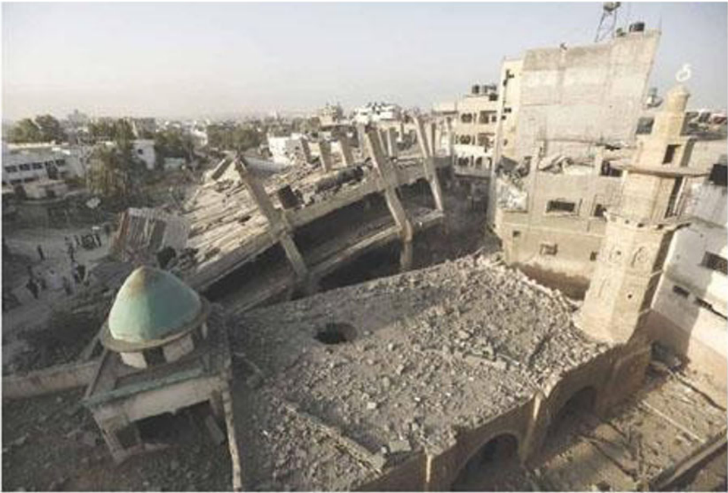
Figure 5. Documentation of damage to the Mohamed Omer Bashir Center at Omdurman Ahlia University.
