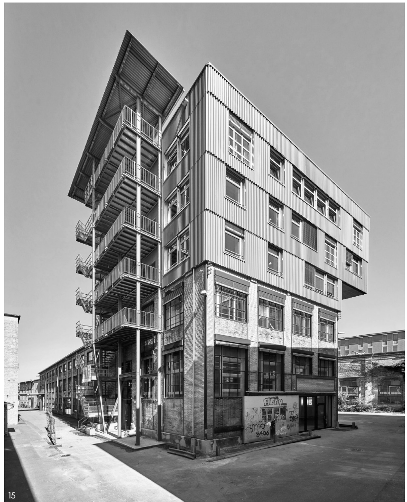
Fig. 15 baubüro in situ ag, K118 – Kopfbau Halle 118, Winterthur, Switzerland, 2017–2021. External view: three new floors added above the existing building, reached via the steel exterior staircase, salvaged from the demolished Orion office building in Zurich. © Martin Zeller, courtesy Zirkular GmbH.
