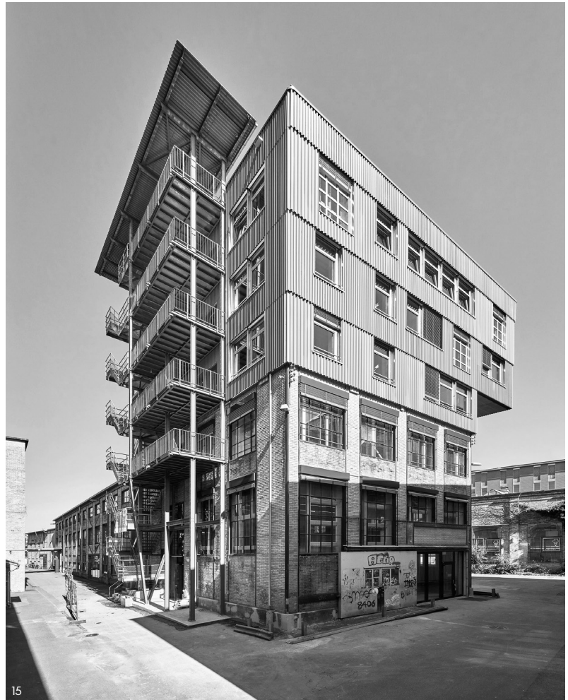
Fig. 15 baubüro in situ ag, K118 – Kopfbau Halle 118, Winterthur, Switzerland, 2017–2021. External view: three new floors added above the existing building, reached via the steel exterior staircase, salvaged from the demolished Orion office building in Zurich. © Martin Zeller, courtesy Zirkular GmbH.
