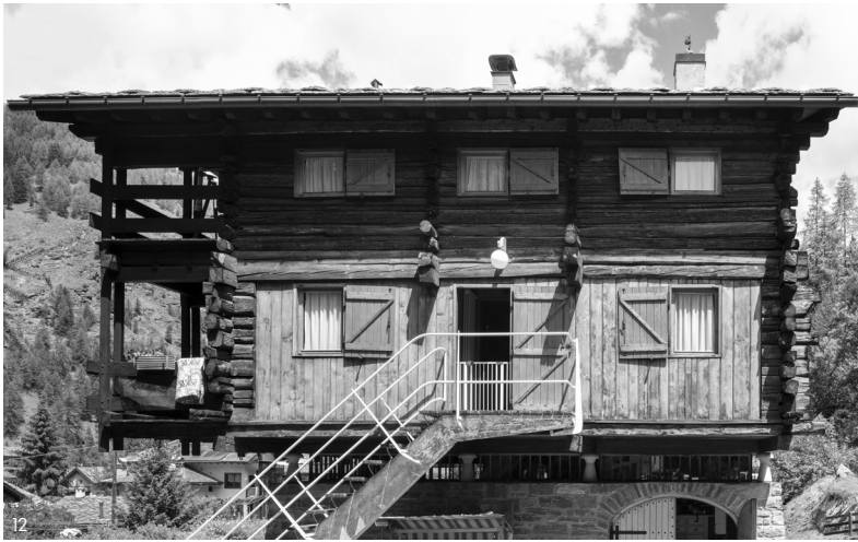
Fig. 12 Carlo Mollino, Casa Garelli, Champoluc, Ayas, Italy, 1962–1965. The south façade with the external access staircase showing the recovered Blockbau structure (in dark timber) and the perimeter wall built with new elements (in light timber). © Davide Franceschini – Altrospazio, 2018.
