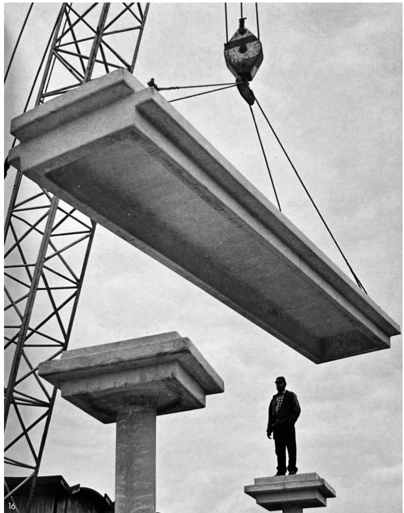
Fig. 16 Assemblage of the “Briona 72” system, front cover of the journal Domus , no. 9 (1977).
