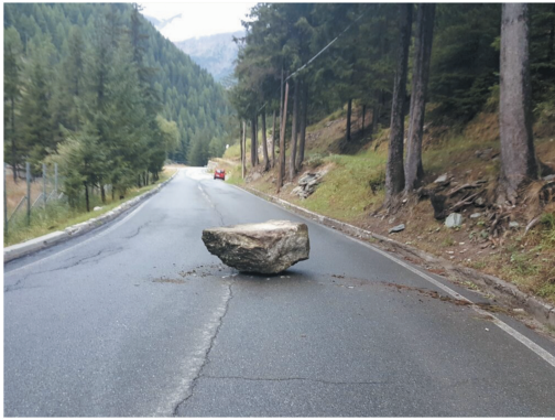
Figure 1. Photo of a rockfall event occurred in Cogne, Italy, on 16 September 2016 after heavy rains. Source: Catasto Dissesti RAVA, F-16-09-2016-00-v-Cm-x.
