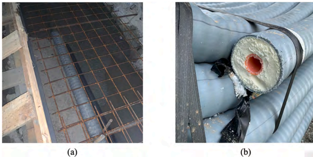
Fig. 11. Jacketed pre-insulated PE-Xa collector pipe: a) positioning within the sidewalk mould and b) cross-sectional view.
