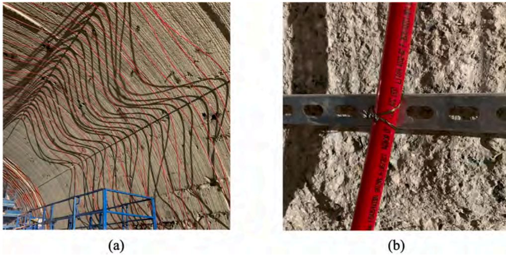
Fig. 7. Pipe pre-positioning through longitudinally wall-attached metal rods: a) view of the left springline and b) detail of the pipe-rod connection with metal wires.
