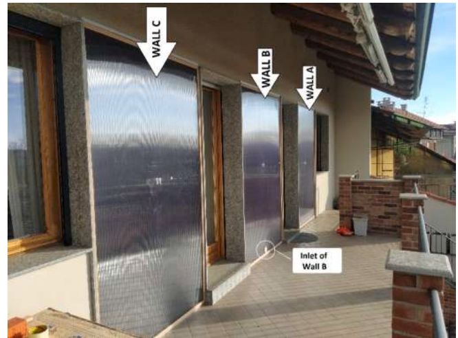
Fig. 3. View of the three full-scale TW modules.
