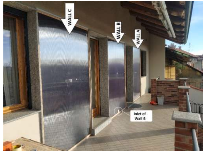
Fig. 3. View of the three full-scale TW modules.
