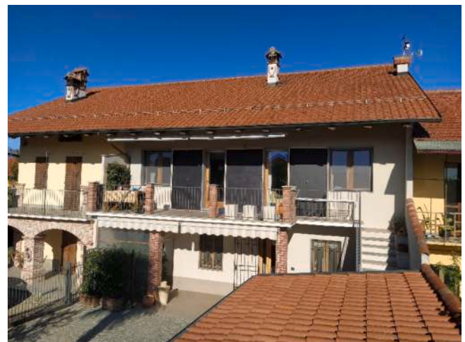
Fig. 1. View of the building and the south-oriented façade where the modules were installed.
