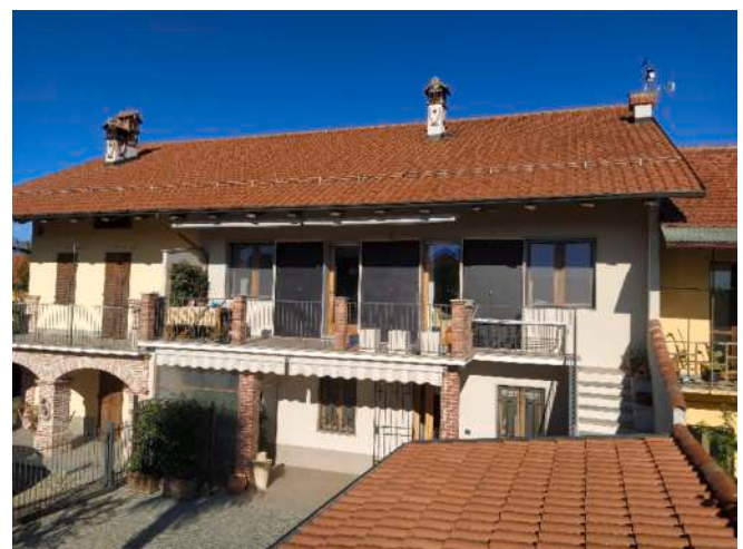
Fig. 1. View of the building and the south-oriented façade where the modules were installed.
