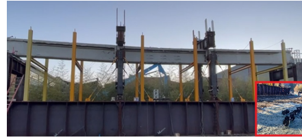
Fig. 4. Real framework testbed: 16 m-long beam from a decommissioned bridge. The bottom-right inset shows the cabling of electric sensors.
