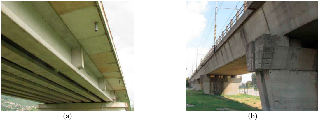
Figure 1: Typical spans for the two case studies: the railway viaduct with PRC girder beams deck, case study A (a) and the one with box girder PRC deck, case study B (b).
