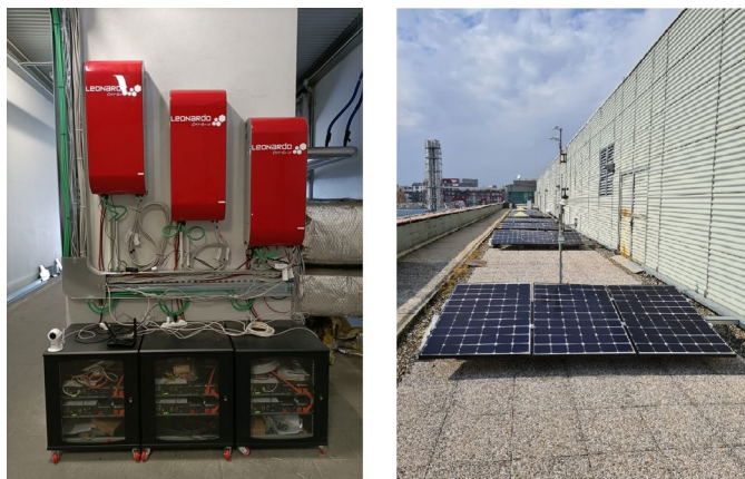
Fig. 2 Real-world equipment of the PVZEN microgrid laboratory. Batteries and inverters (right side), and PV panels (left side)
