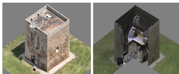
Figure 1. UAV photogrammetry (left) and terrestrial laser scanning (TLS) data (right). (Editing: E. Pupi)
