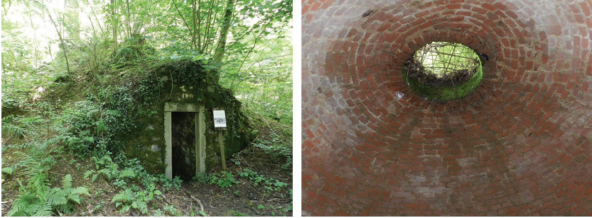
FIGURE 6 Ice-House in the Woods near Ronco Biellese (left); Opening in the Ice-House Ceiling (right, used to draw ice during the summer)
