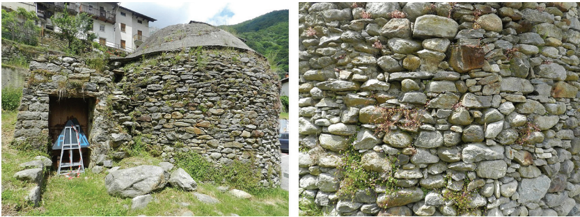
FIGURE 7 The Ice-House in Piedicavallo (left); A Detail of the Stone Masonry (right)
