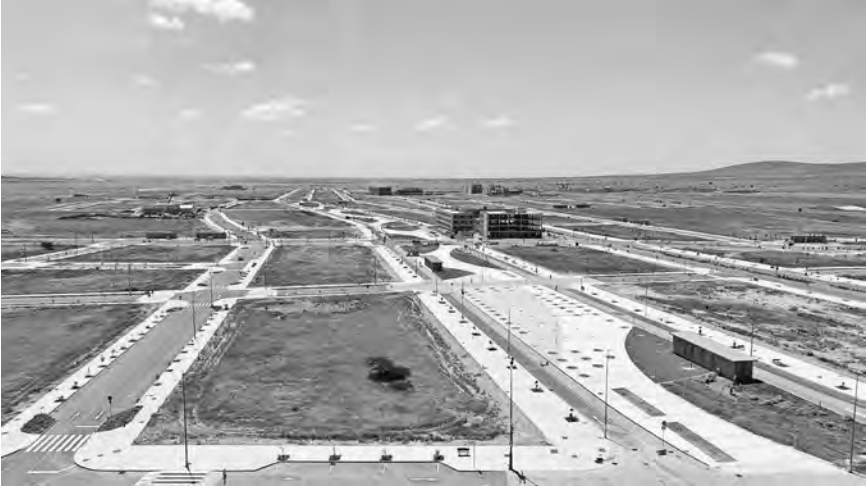
FIGURE 2. An aerial view of the construction site of Konza Technopolis. Photo by author.
